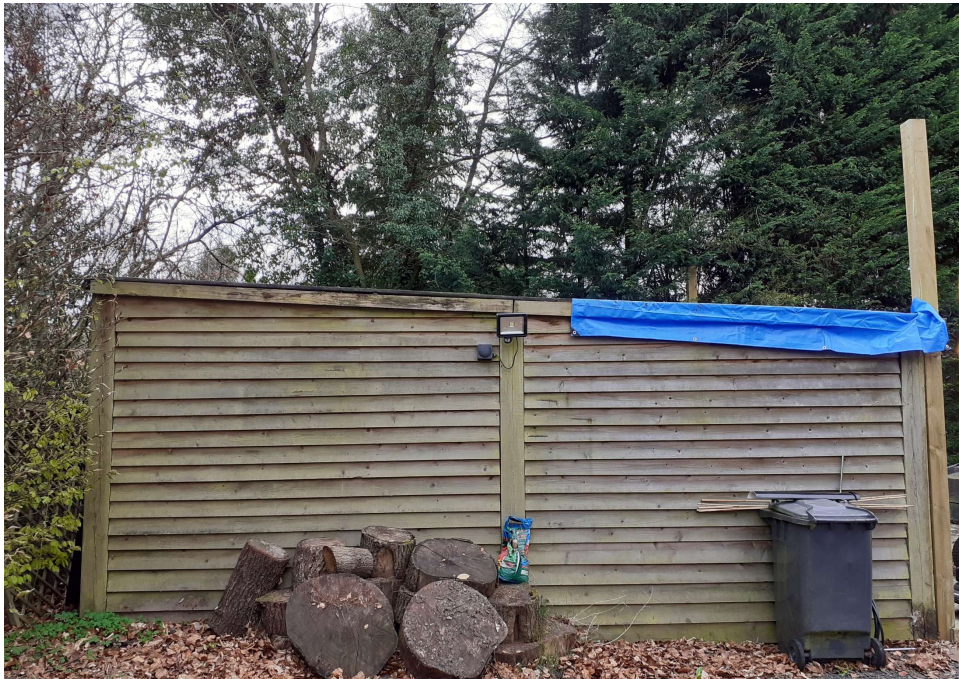
East elevation of existing storage shed
